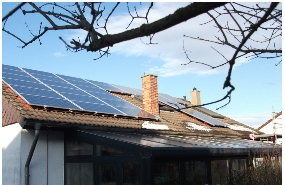
The photo shows how the SolarEdge system allowed Mr. Schneider to install modules close to the chimney without risking disproportional energy losses.
